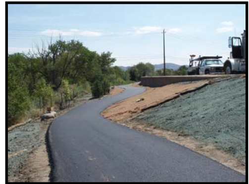
Reno-Sparks Indian Colony Floodwall and Levee
